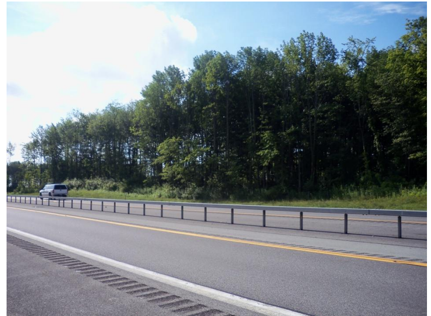
Route 840 – View East
